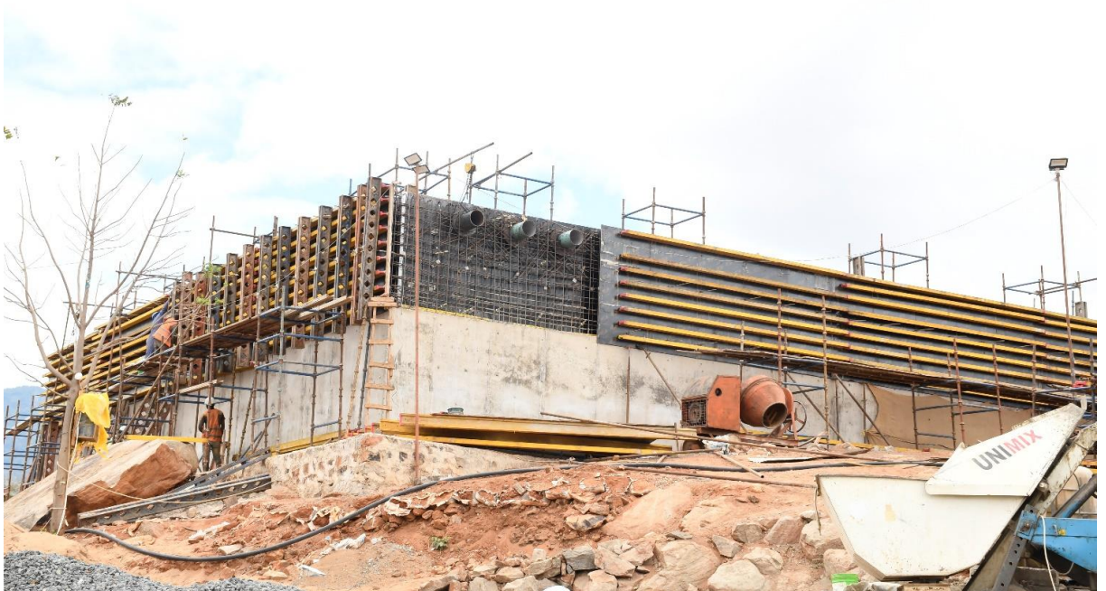
Tank la Mradi wa usambazaji maji Babati Mjini, 2023
